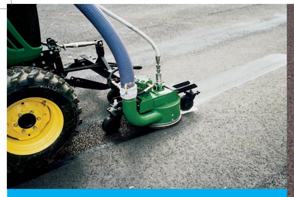
In the U.K., High Pressure water jetting has long been a reliable method for removing excess binder on fatted-up roads and for cleaning contaminates from surfaces (oil on roads, chewing gum on paths etc.).
